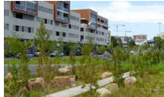
Figure 127: Low Impact Stormwater Design - Bioswales
